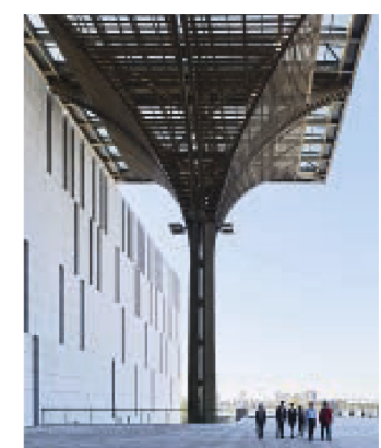
Das Binhai Cultural Center in Tianjin (CHN).
